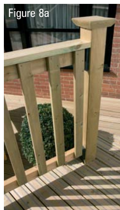
Figure 8a: Strength assessed raised level parapet system. Figures 8b and 8c: Contemporary design modular systems for raised decks
